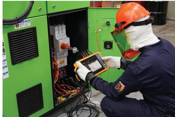
A Fluke 1777 Three-Phase Power Quality Analyzer in use. Power quality analyzers are one of the necessary types of tools for troubleshooting power quality problems.
