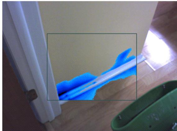
When insulation has settled over time, is missing, or damaged, a thermal camera can often pick up a different thermal pattern compared to the rest of the wall. These areas can often be a source of heat loss or gain, and, if bad enough, can lead to significantly higher energy usage.
